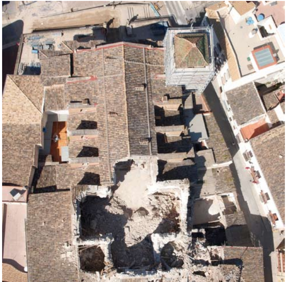
Figure 1. The condition of the church of Santiago in Lorca after the earthquake of 11 May 2011.
