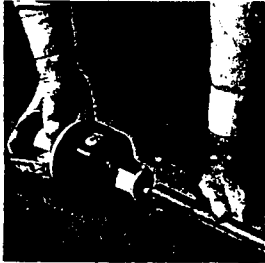
Tubing is placed inside ferrule and nut assembly that has been pre-assembled on Hydraulic Swaging Unit.
