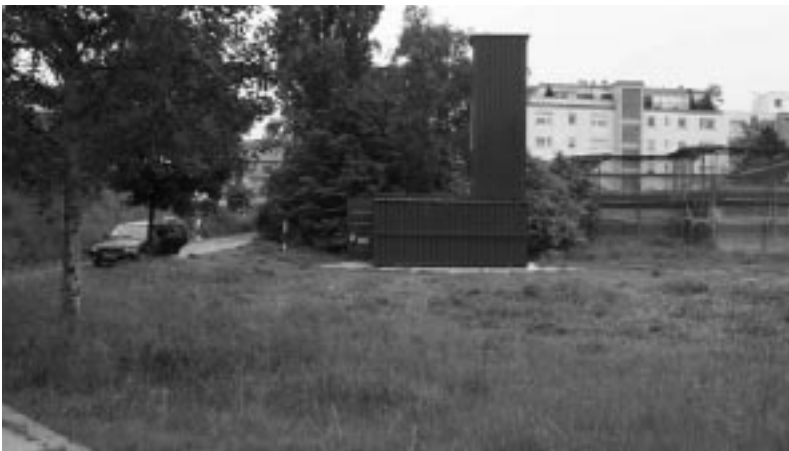
Groundwater remediation plant
